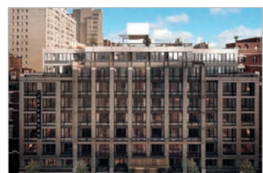
211 EAST 13TH ST 88 units New York, USA
