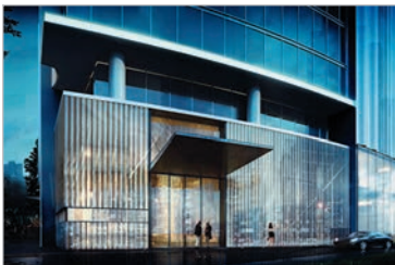
ARABELLA 100 units Houston TX, USA
