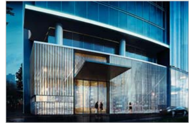
ARABELLA 100 units Houston TX, USA
