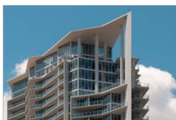
SIGNATURE 246 units St. Petersburg, USA
