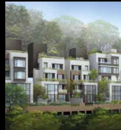
MOUNT KELLETT ROAD, HONG KONG / 13 UNITS
